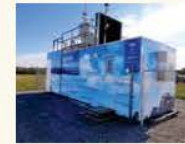
N7 Air Quality Monitoring Station
