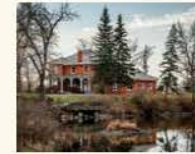
P6 Walker House + grounds
