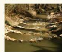
S8 Fish passable weirs (No public access)
