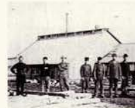
P2 Sawmill covered structure
