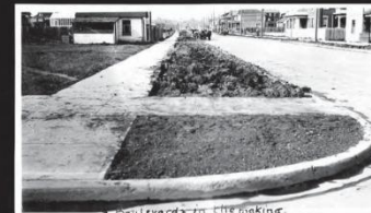
Boulevard in the making
