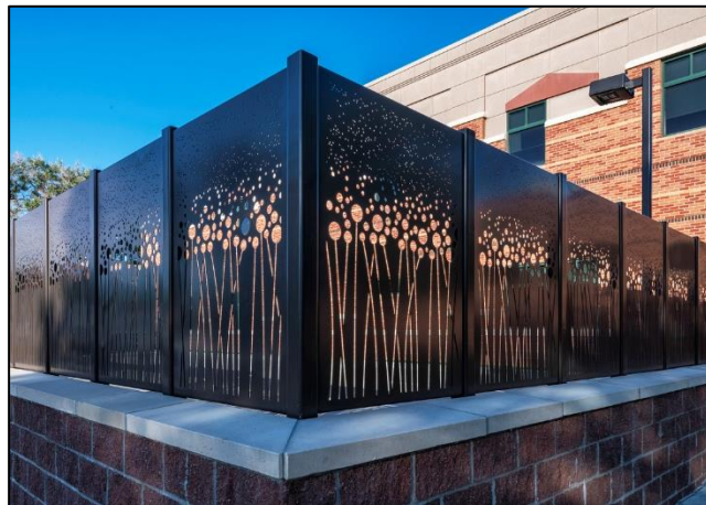
Decorative metal screening of at grade mechanical equipment.
