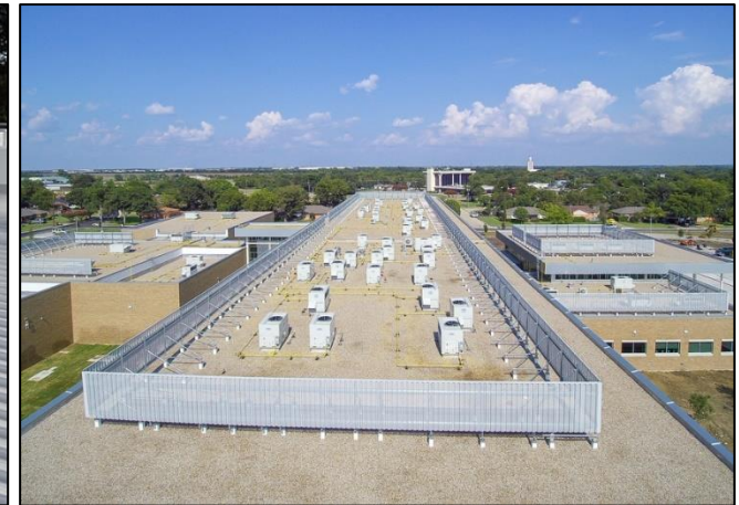
Screening a large area of rooftop equipment with metal rooftop screens.
