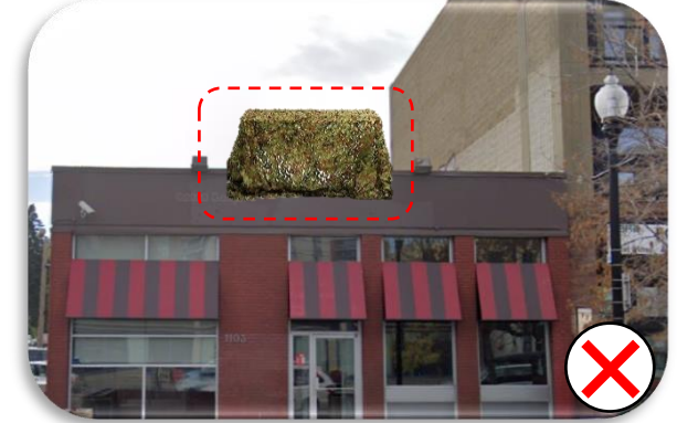
The attempted camouflage is not harmonious with the building and does not conceal the equipment.
