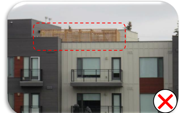
Screening should blend into the building design, rather than draw pedestrians' attention to the screen.
