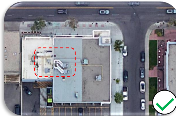
Equipment is located central to the rooftop, not visible from public spaces, houses or apartments.
