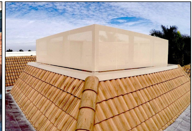
Screening of rooftop equipment with coloured awning fabric that is consistent with the building form and finish.
