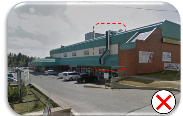
Equipment should be located out of view of public spaces, otherwise camouflaged or screened.
