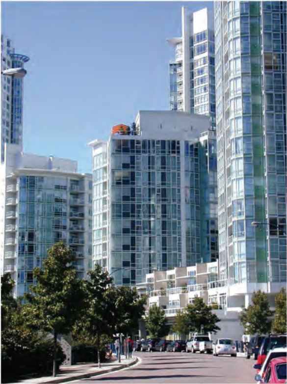
NORTH FALSE CREEK, VANCOUVER, BC Podium (3 storey) street wall and slim towers above
