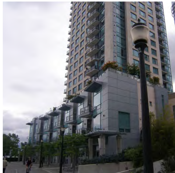
Stepping back the tower to define the building podium and the street walls. This also reduces the negative impacts of taller building parts on the adjacent streets and surrounding context.
