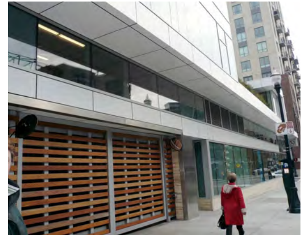
Use attractive vehicular entry doors at a street frontage.
