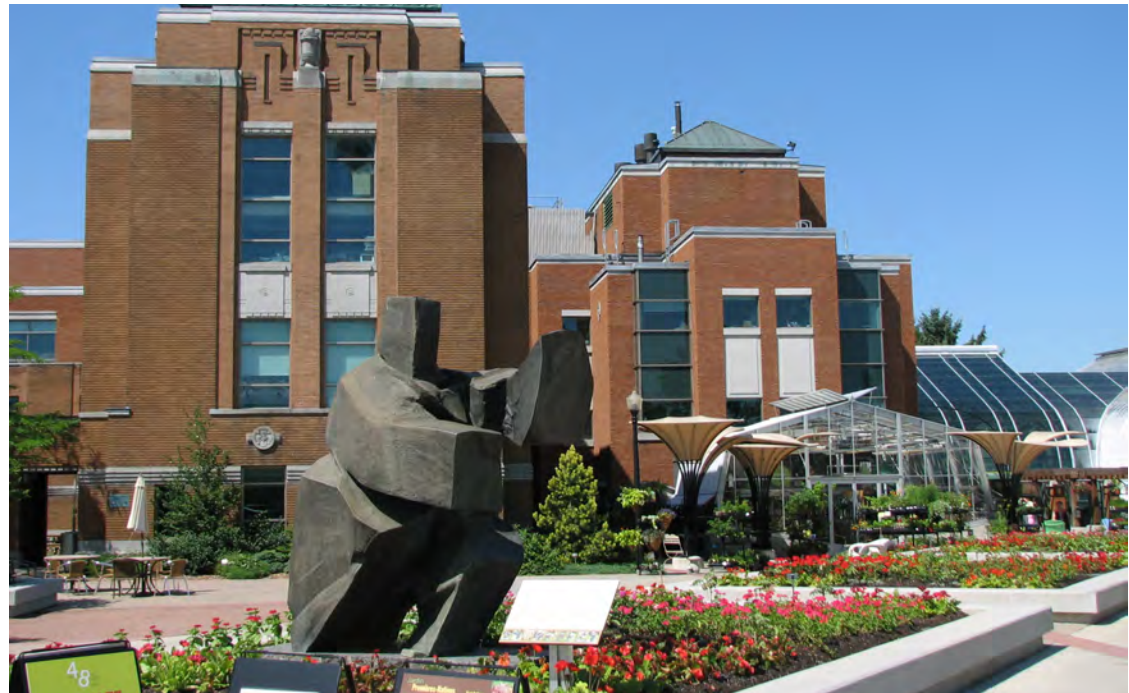
Locate open space for gathering people at sunny locations that offer optimum sun exposure.
