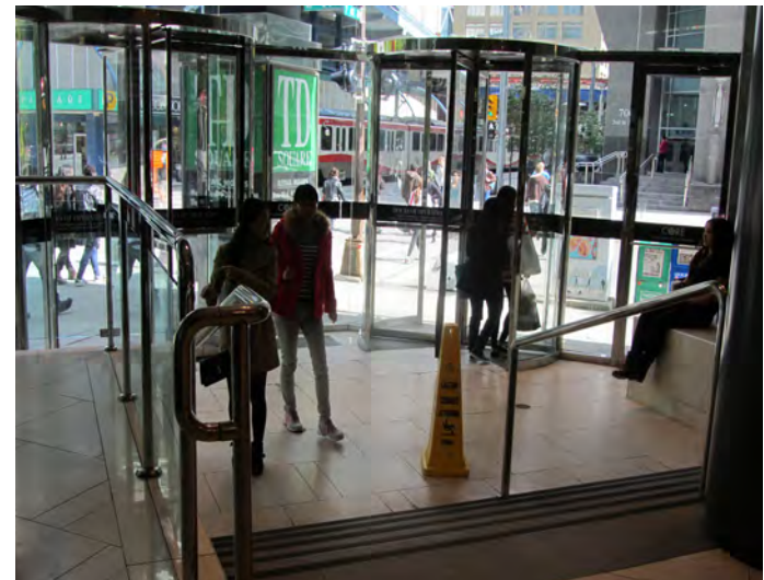
In areas requiring floodplain considerations, accommodate shop access through the careful design of stairs and/or ramps within the building or tenancy.
