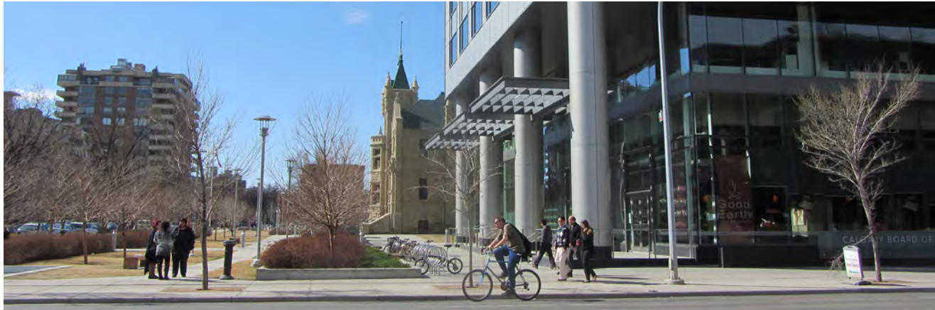
Colonnades providing sun access to the internal facade by having a 2:1 height-to-width ratio like 3.0m:1.5m. For high colonnades, provide canopies no higher than 3.0m in height, to protect pedestrians from weather elements effectively.
