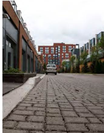
Permeable pavers at a lane with well-vegetated edges and gardens, all part of a sustainable drainage system.
