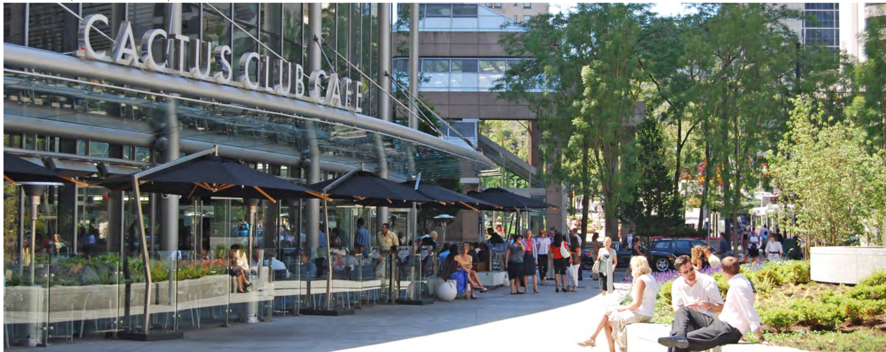
Animate corner plazas with active uses to provide a comfortable and safe pedestrian environment.
