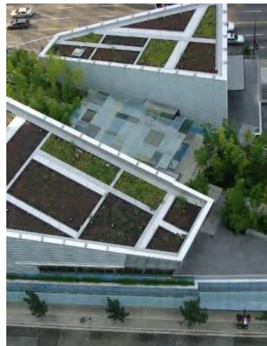
Landscaped roofs and roof gardens save energy while adding landscaped amenity space for building occupants.
