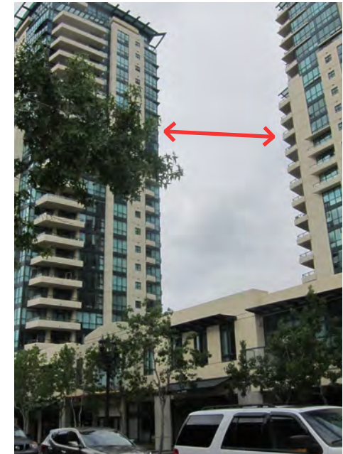
Keep towers separated at a minimum of 24.0m to maximize privacy and sun access.
