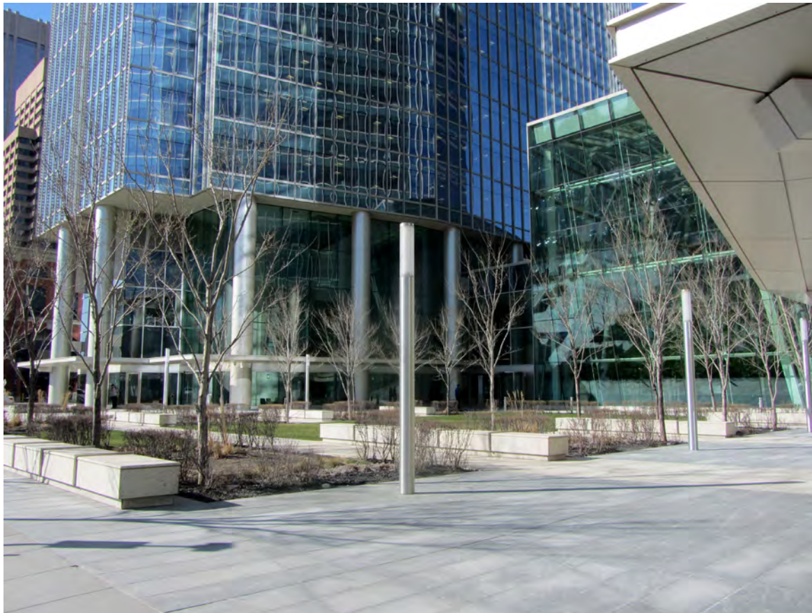
Design buildings with careful setbacks and tower placement to ensure sunlight access to on-site open spaces.
