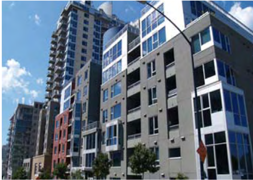
Use a street wall ratio of 1:1 for a location that has a high intensity of use such as this multi-residential development.
