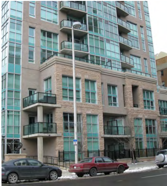
Residential podium (or base building).
