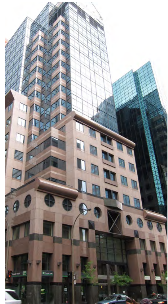
A commercial podium with colonnade at the ratio of 2:1 and a street wall height to street width ratio of 1:2. The step-backs at the upper building parts help to mitigate adverse shadow impact on adjacent public realm, sidewalks and surrounding building facades.
