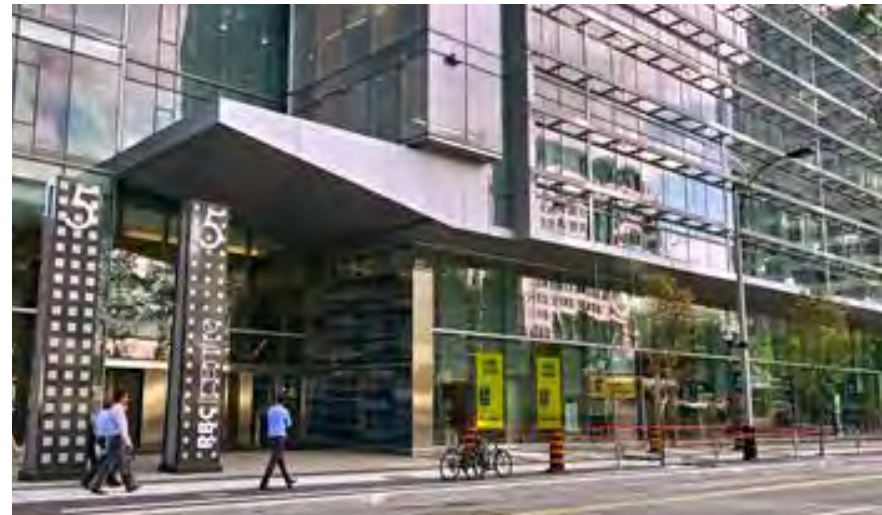
A retail street frontage with a fine-grain rhythmic repetition of active uses, multiple shop and lobby entrances, all oriented towards the street.
