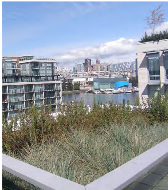
Native vegetation on landscaped (or green) roofs reduces water use, solar gain and adds amenity space for residents.
