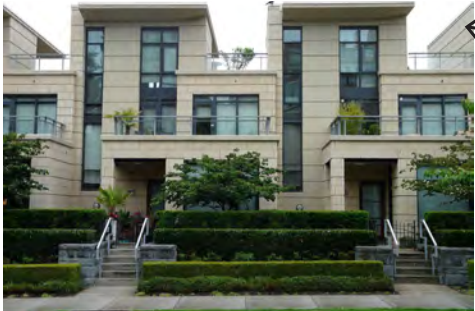
Landscaped setbacks with grade separation from sidewalks to enhance the privacy of residents.
