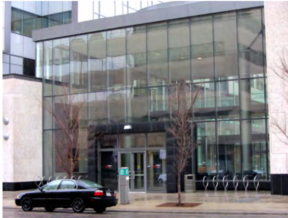
Integrate on-site bicycle racks with the design of the building envelope at ground level.
