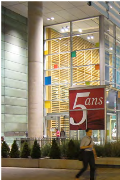
Easily distinguishable building entrances.
