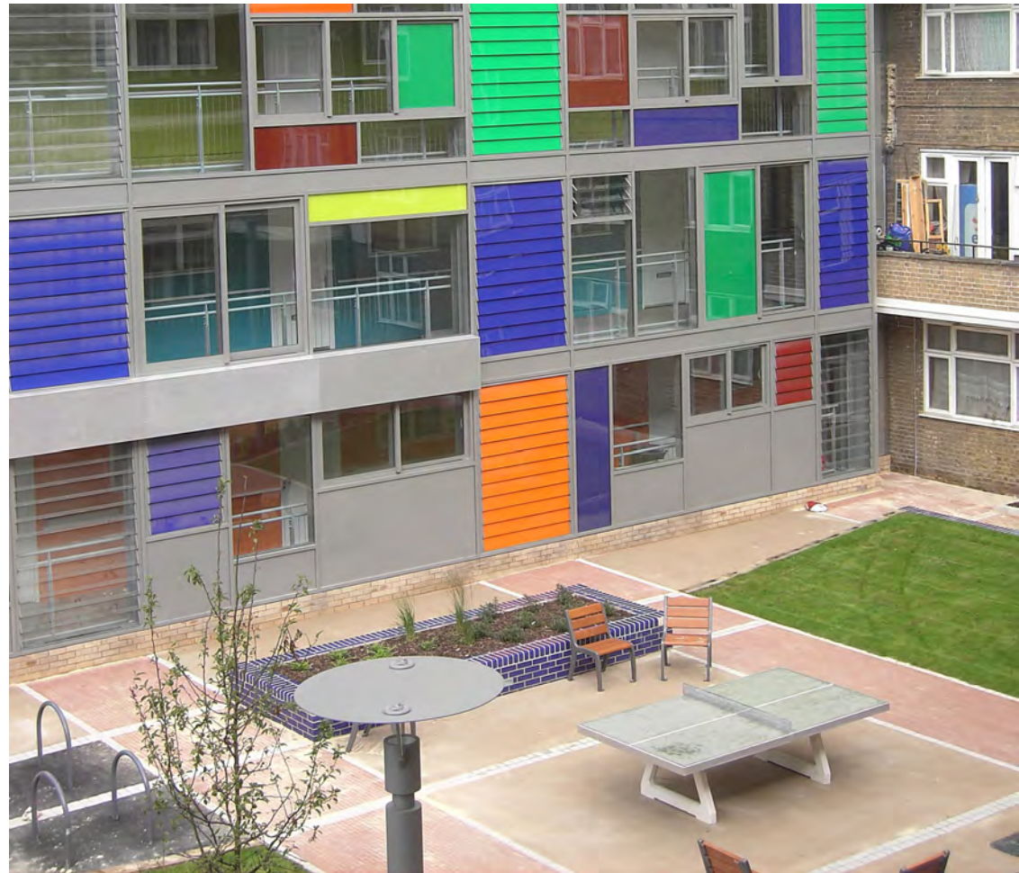
The overlooking of private and community green amenity allows for natural surveillance and increases the sense of safety and security of its users.
