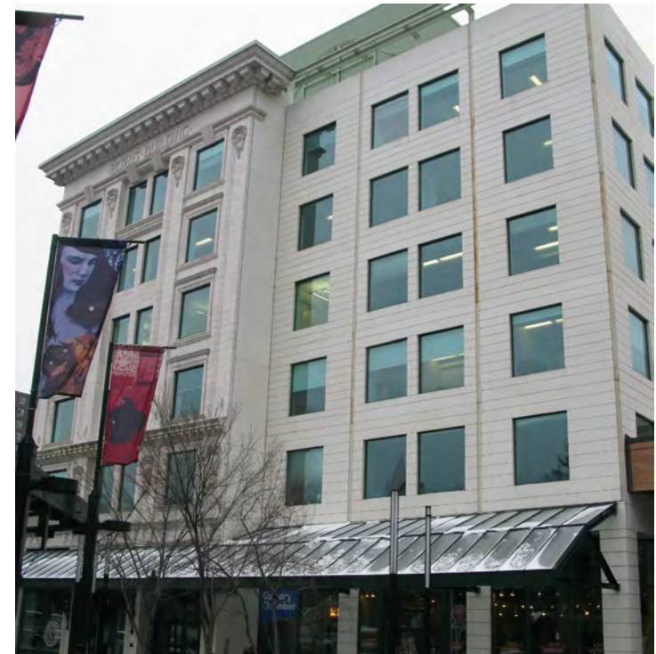
This contemporary development is respectful of the adjacent heritage building to its left, using compatible fenestration (or window treatment), cornice lines, awnings and cladding materials.
