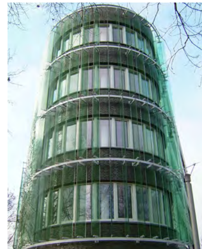
Use a controllable glass louver shading system to reduce solar heat gain and cut down cooling costs in summer, while maximizing the use of natural daylight.
