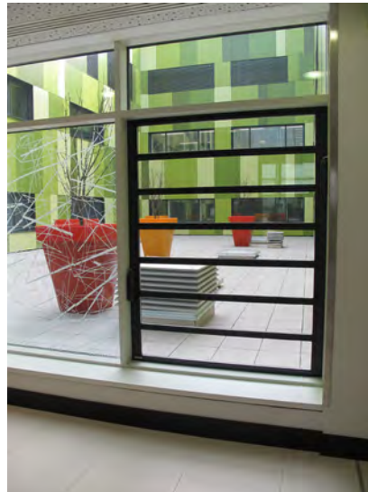
Natural ventilators at courtyards and operable windows aid in efficient resource use.
