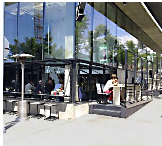
A sensitive treatment using gently sloped ramp and clear step placement at a street corner to accommodate grade change.
