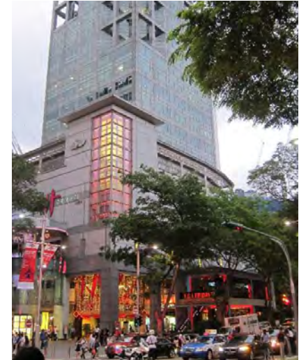
A good corner building design treatment showing emphasis of building corner, through the use of colours and transparency in the facade treatment. Such design treatment activates and promotes building corners as sites for people to gather and socialize.
