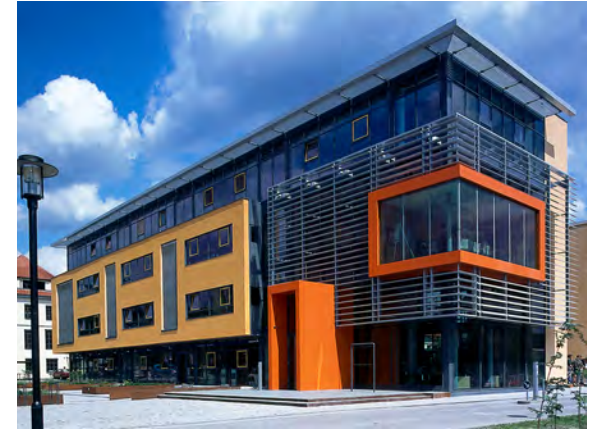
Use a wrap-around wall treatment with interplay of materials and accent colours to reduce bulk and add fun to a building facade.
