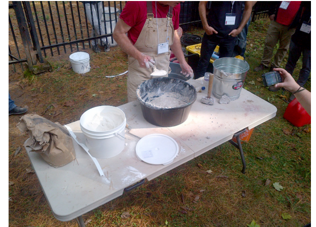
Master stonemason mixing lime mortar at historic masonry workshop. Montebello, QC, 2017
