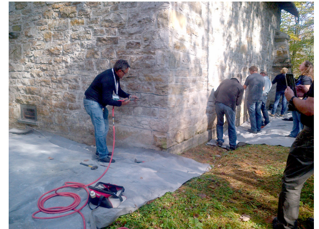
Heritage architects and stonemasons raking out and repointing mortar joints. Montebello, QC, 2017
