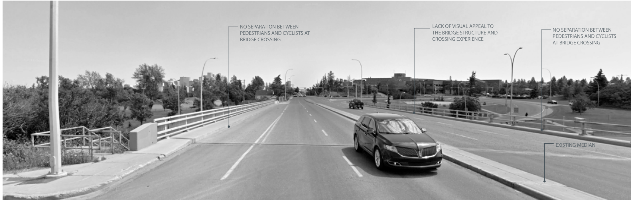
Figure 3.18 Existing Condition at Crowchild Bridge
