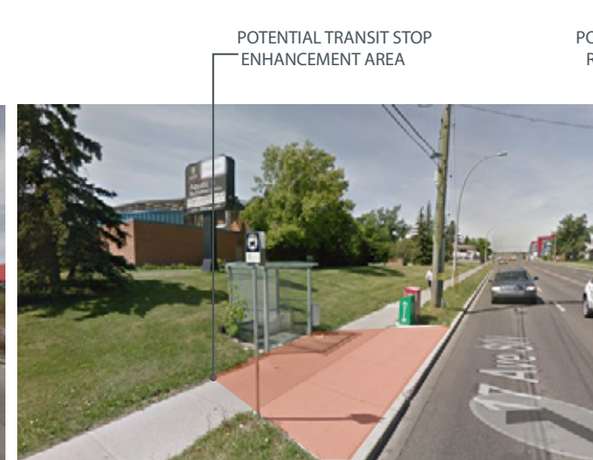
Figure 2.17-3 Covered Transit Bus Stop at The Corner of 29 St SW, South Side
