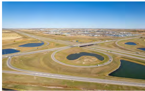
CANAMEX Corridor interchange nearby at Stoney Trail and Glenmore Trail S.E.
