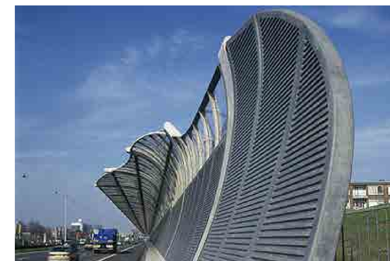
Cantilevered wall with solar panel
