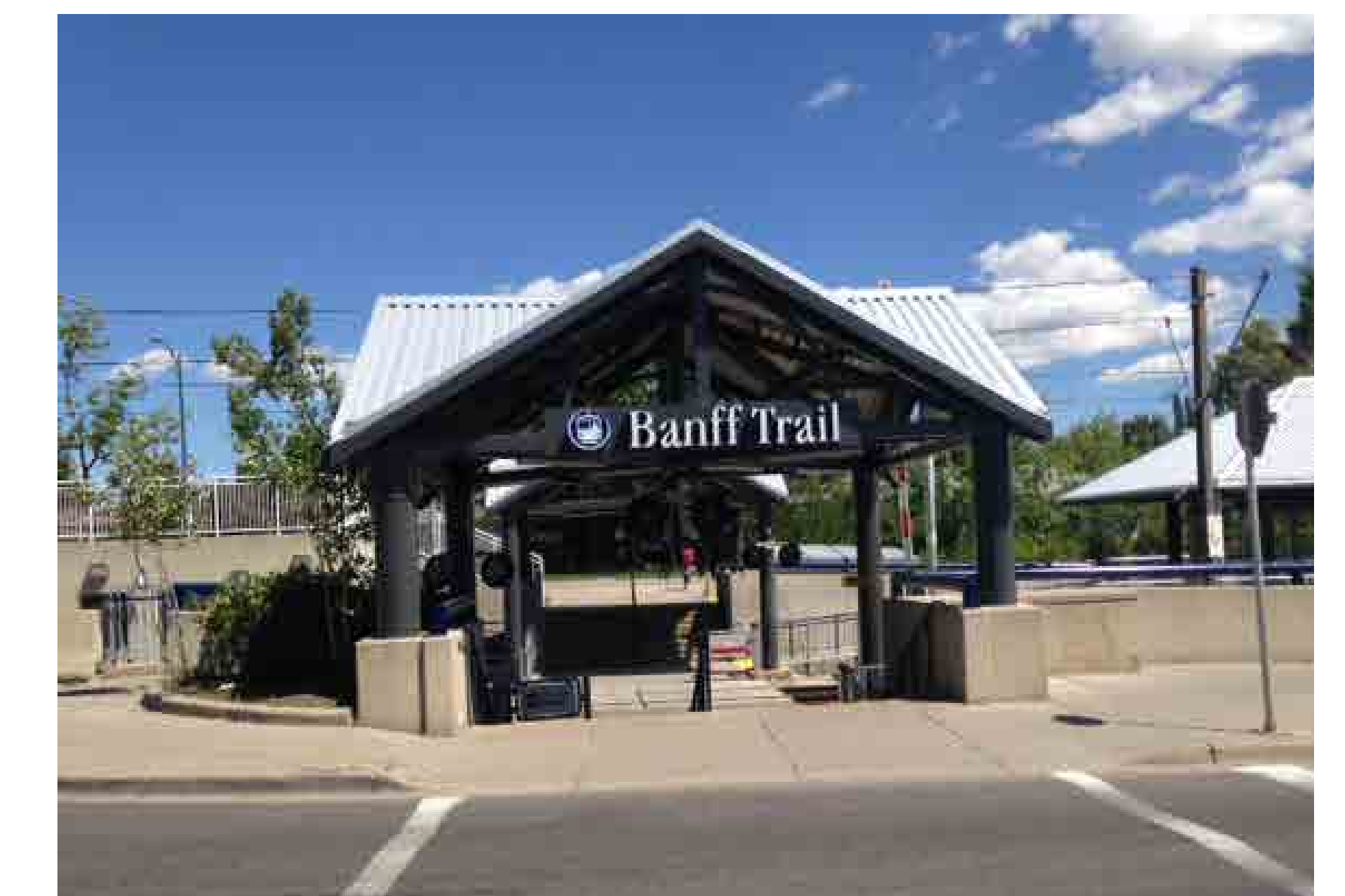
Banff Trail LRT station
