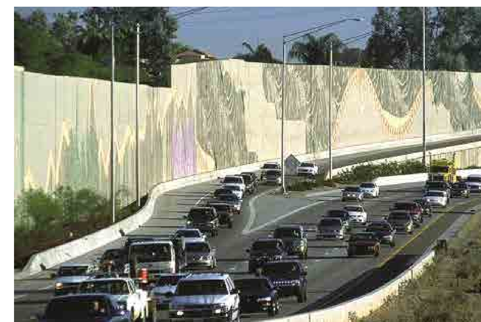
Custom panel wall
