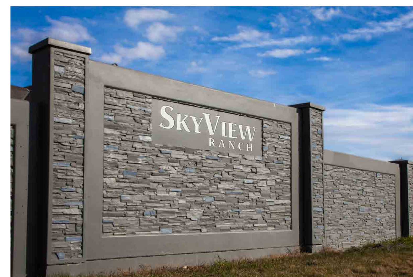
Custom panel wall
