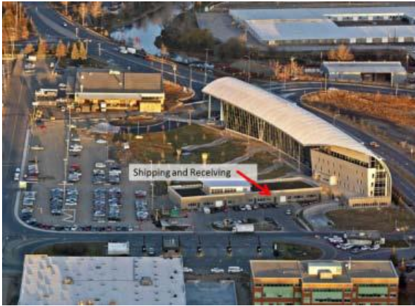
The Water Centre
