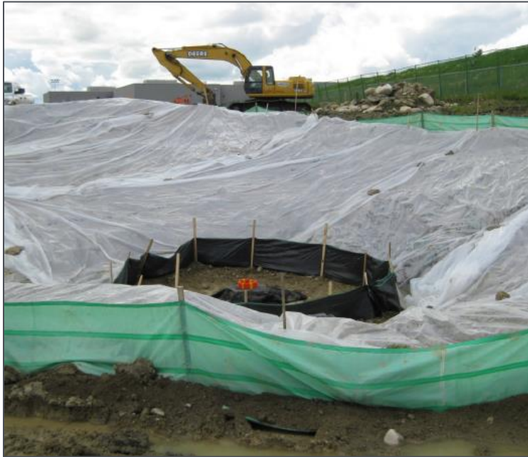
Photo 3 Isolation Measures, Poly Sheeting
