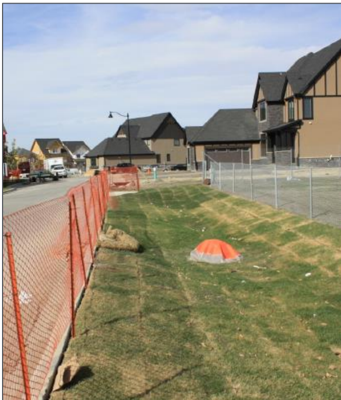
Photo 4 Temporary Sod Cover
