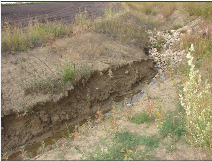
Photo 8 Channel Erosion
