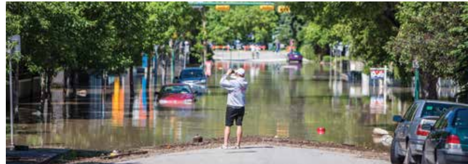
ENMAX substation #32 surrounded by floodwaters.
